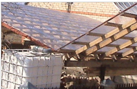
Fig. 4. Rain water collection system
