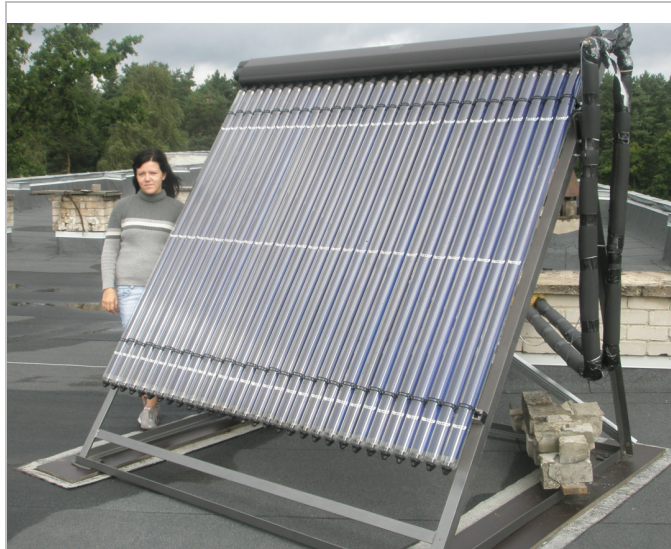
Fig. 2. Solar energy collector Vitosol 200 SD 3 m 2 on the roof of the building in Ulbroka
